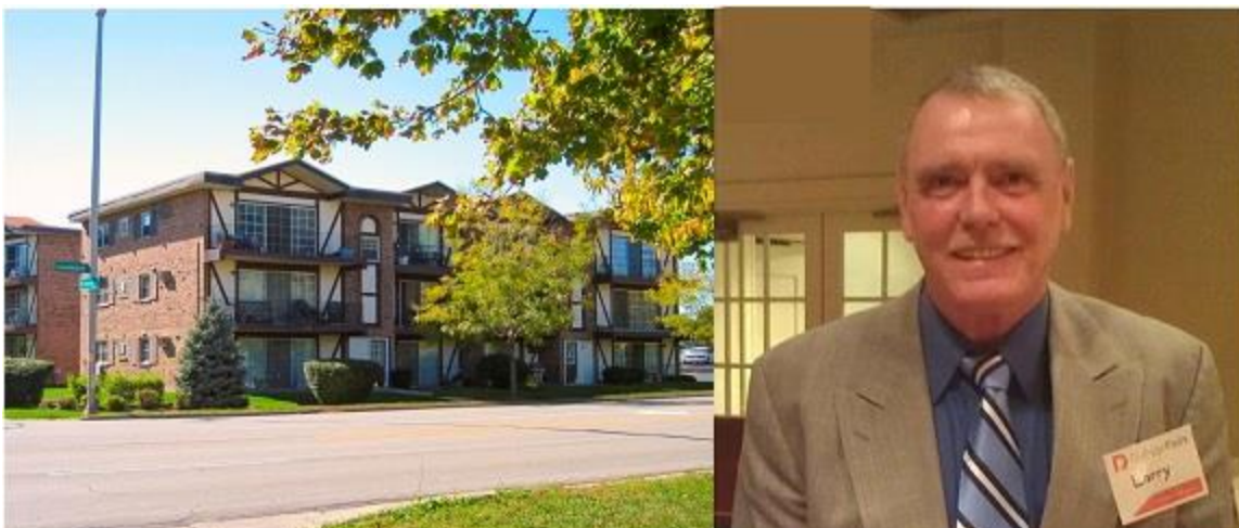
Left: Supportive Housing apartments at Olympus Place in Naperville for DuPagePads program participants.
